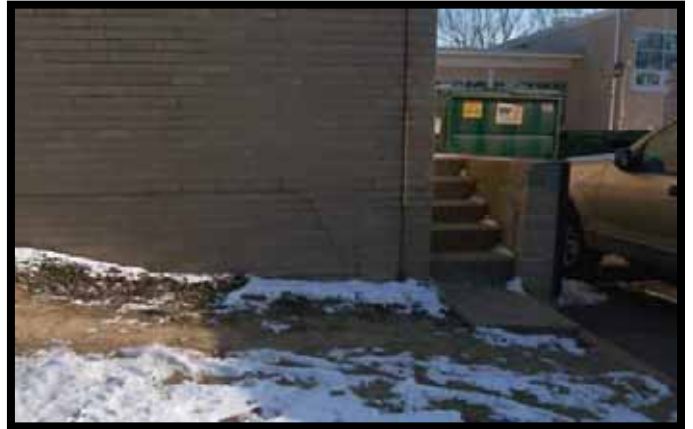
Cracking at Loading Dock
