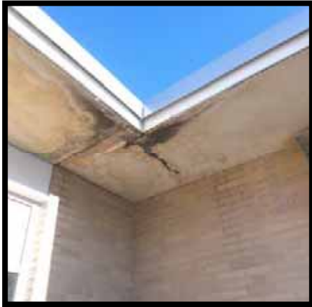
Soffit Damage
