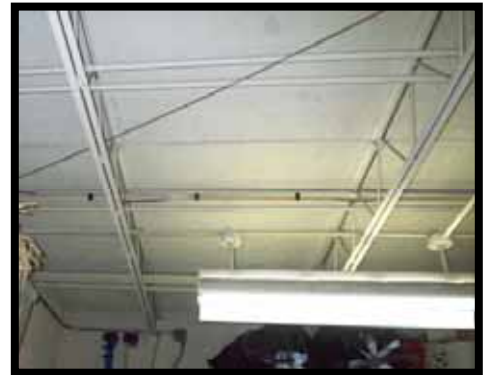
Existing Tectum Decking & Steel Joist system
