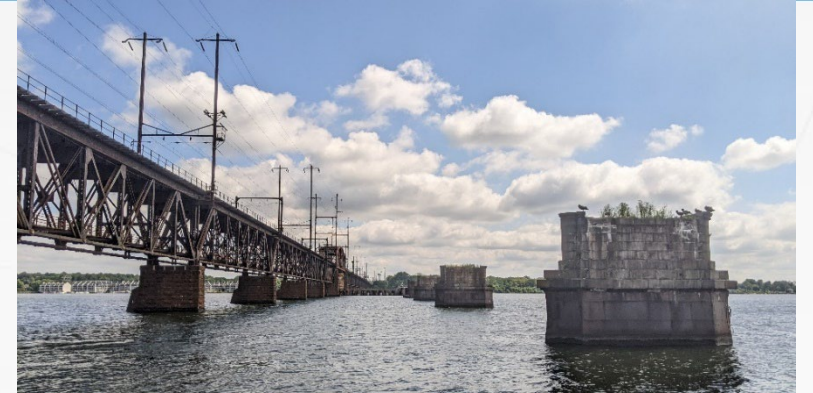
The 1866 remnant piers adjacent to the existing Susquehanna River Rail Bridge
