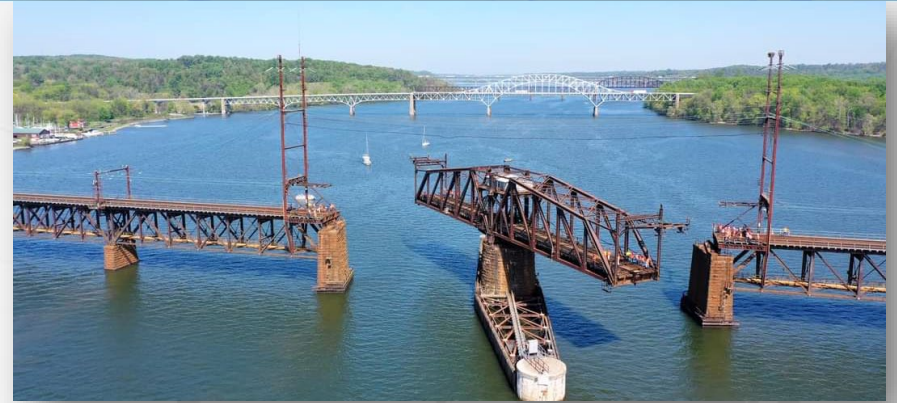
Susquehanna River Rail Bridge opening for marine traffic.
