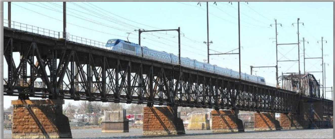
Train crossing Susquehanna River Rail Bridge
