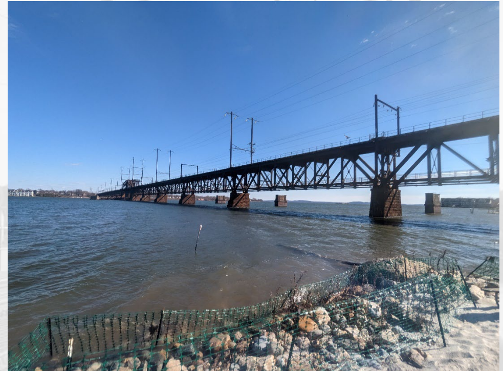
Susquehanna River Rail Bridge & shoreline
