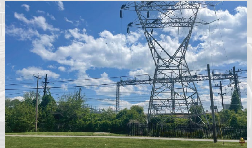
The existing BGE tower located across from Rodgers Tavern in the Town of Perryville, Maryland.
