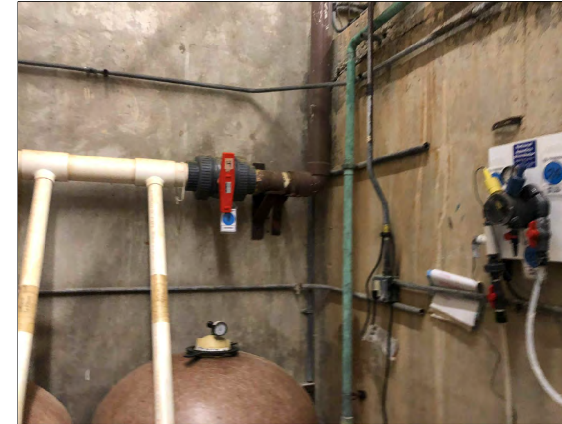
1 E-1.01 EXAMPLE OF ABANDONED PIPE TO BE DEMOLISHED SCALE: NONE
