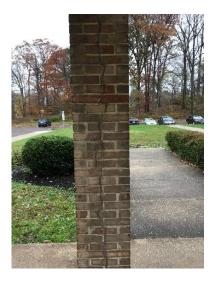
• There are a couple of loose bricks over top of piers at the cafeteria. This is probably due to thermal expansion of the steel members that bear on the masonry piers.
