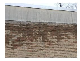
• Some joints have exposed horizontal reinforcing that has begun to rust. This is probably due to the moisture issue. The rusting action causes the reinforcing to expand and crack the mortar in the joints.
