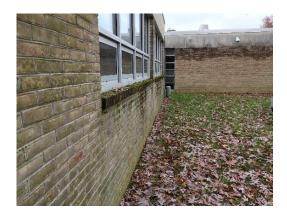
• Damaged and eroded brick joints was noted especially at the top sections of the wall where there is evidence of moisture. The constant moisture has probably softened and has caused the joints to deteriorate.
