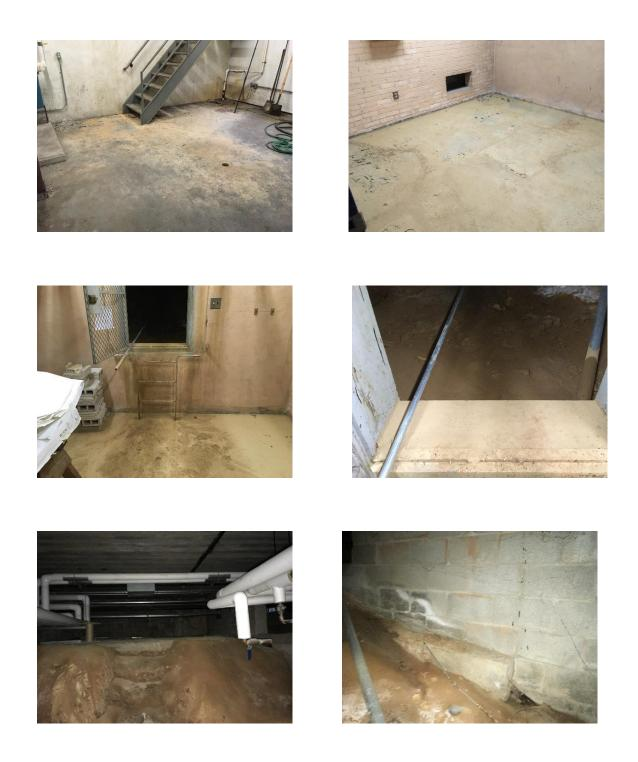
• Signs of water infiltration into the main mechanical room at the bottom of the boiler stack. Water appears to be collecting inside the stack and then coming thru the bottom of the stack wall. The water has begun to rust some of the adjacent pipe supports.
