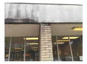
• Typically, there are signs of moisture along the upper sections of most of the exterior walls. The cause of the moisture is unknow, but it could be from water spilling over from the roof.
